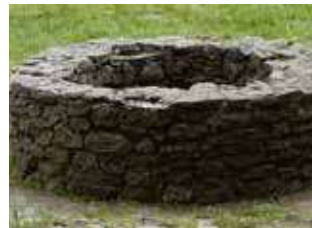
Drainage in wells
